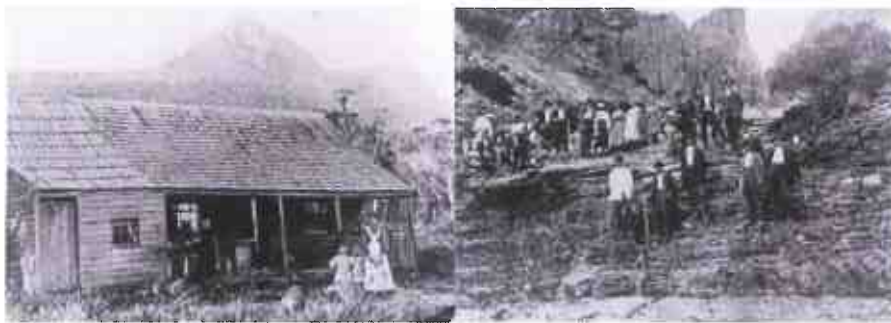
Life at Storys Creek early in the 20 th Century: (left) a shingle-roofed miner's cottage; (right) a picnic party on Stacks Bluff.
