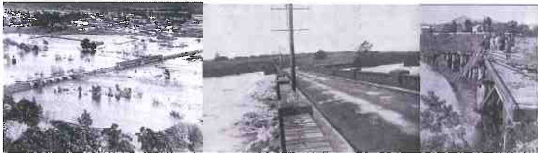
(Left) The viaduct and South Esk Railway Bridge at Longford during the 1929 flood. (Centre) The Perth Road Bridge resisting the South Esk River shortly before it was swept away. (Right) Flood waters tear the railway line off the Avoca Railway Bridge.
