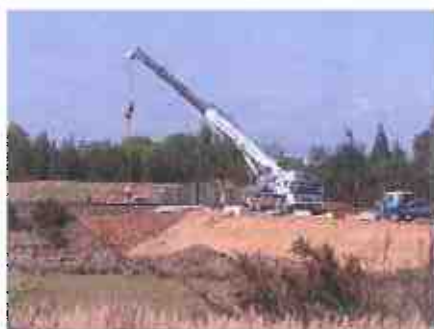
Longford levee bank construction
