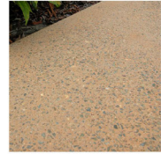
Exposed coloured concrete pavement.
